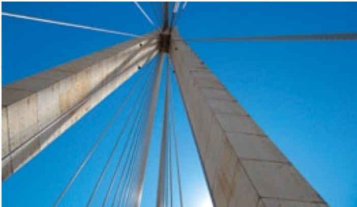
A suspension bridge was all cables, concrete and elegance.
